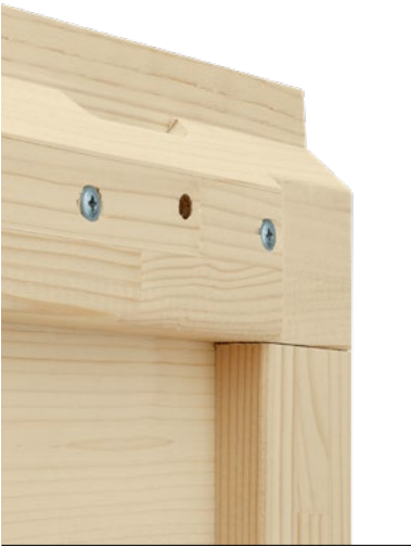
Reinforcement at section ends
